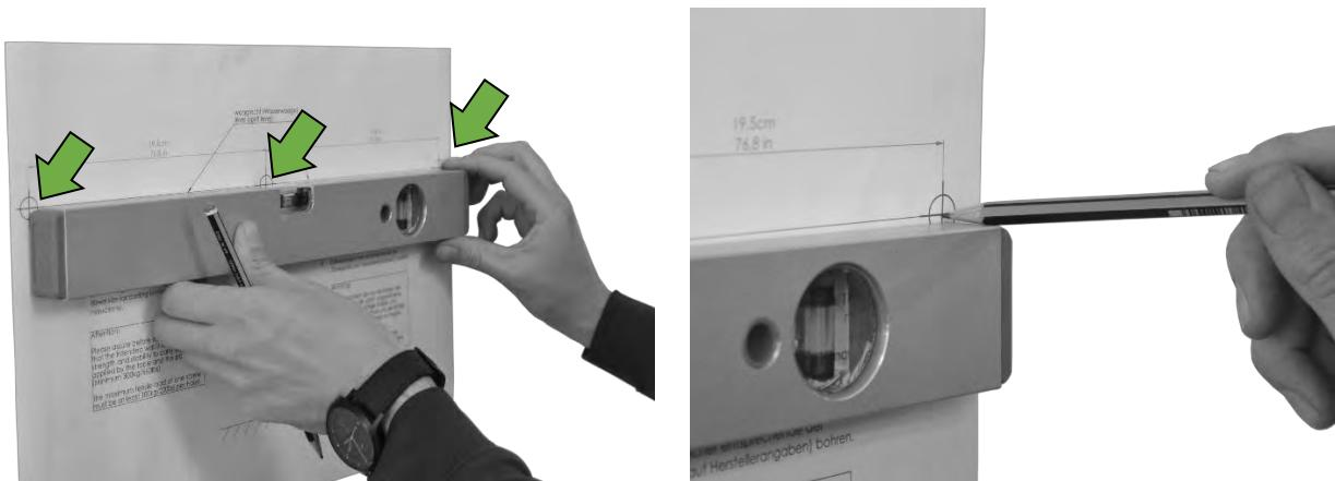
After the three necessary drill holes have been marked, these are to be drilled with a proper drill bit suitable for the designated wall. The drilled holes must then be cleaned accordingly and freed from dirt.
