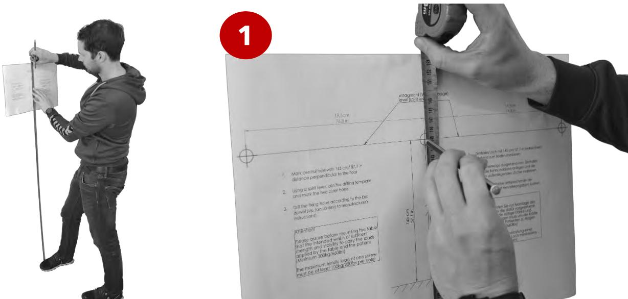
Then, with the aid of a spirit level, mark the two holes indicated on the outside of the drilling template horizontally, each 19.5 cm (= 76.1 inches) apart from the center hole.
